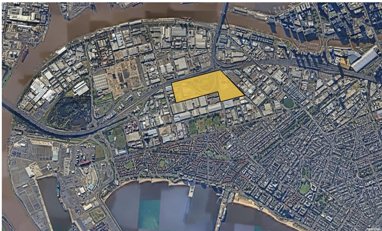
Figure 6 – Approximate extent (orange) (Source: nearmap 2020)
