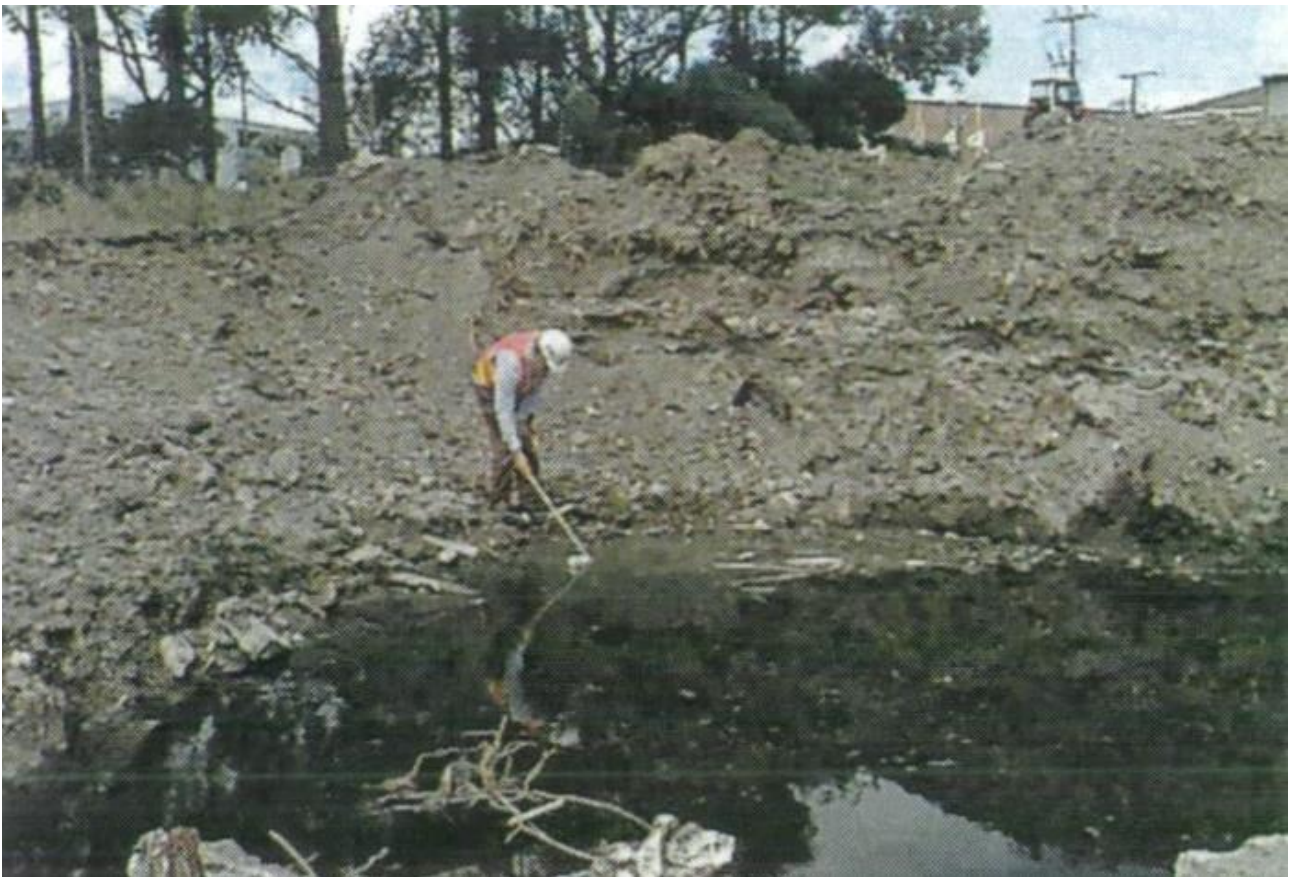
Figure 8 – Leachate impacted water being sampled with waste clearly visible. (Source: Baulderstone Horibrook Engineering 1996)
