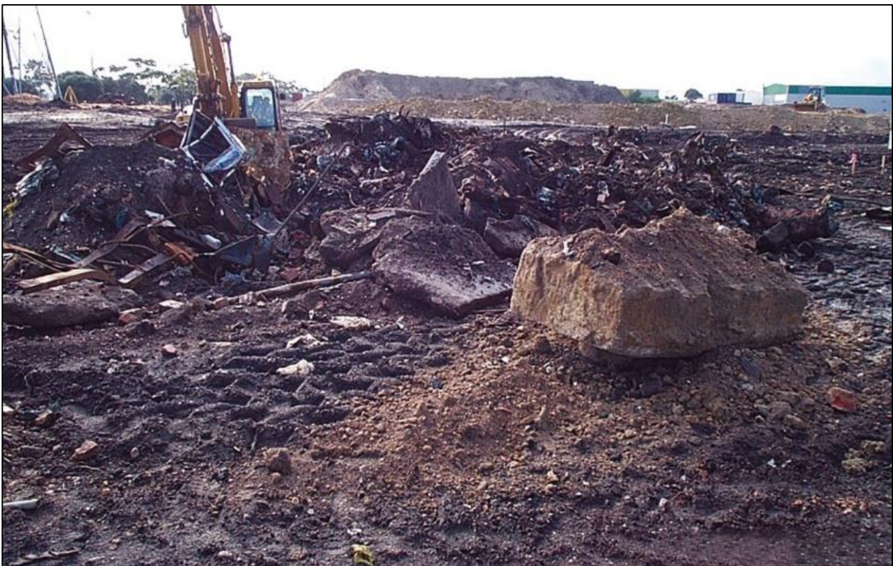
Figure 13 – Exposed waste during 2001 capping works at Port Melbourne Tip - South (Source: Australian Turfgrass Management 2005)
